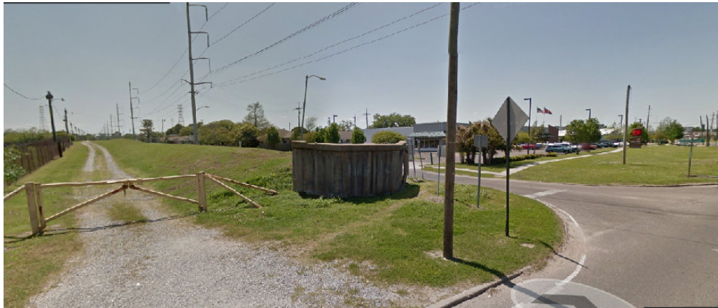
l. Looking Southeast, from Jefferson Hwy, Levee
