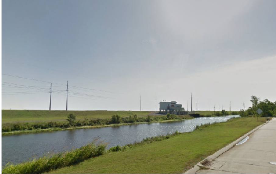
Figure 7.8. 40 Arpent Canal, Levee/Floodwall, and Bayou Villere Pump Station Google Earth
