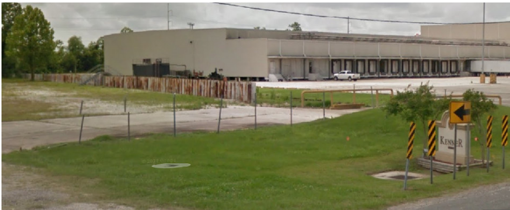
c. Looking South from Airline Hwy, Sheet Pile
