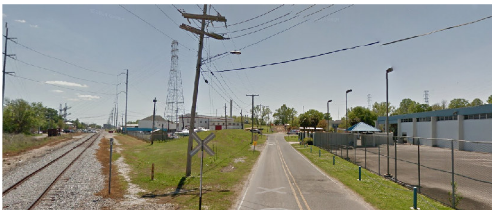
p. Gaps at Public Belt Railroad and River Rd
