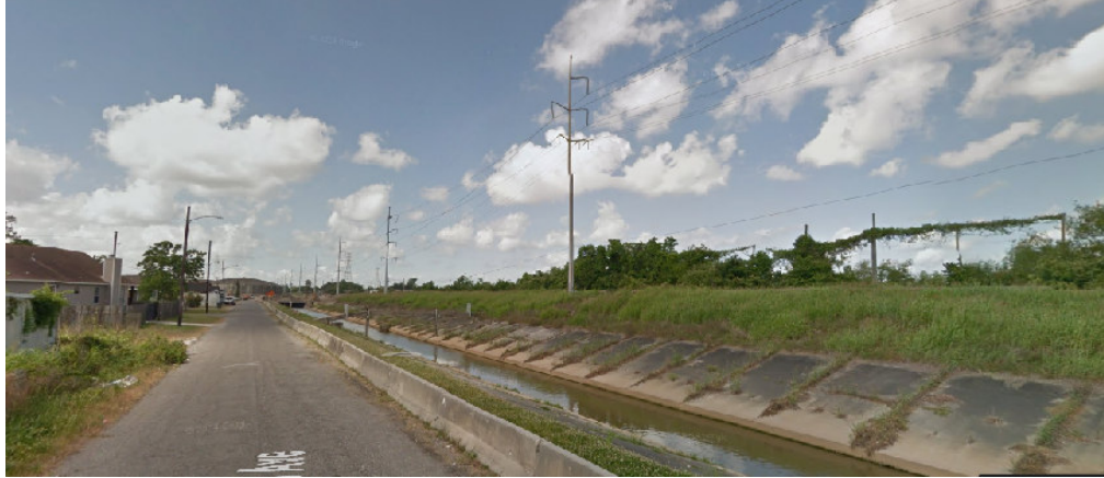
k. Looking South, from Earhart Expressway, Levee
