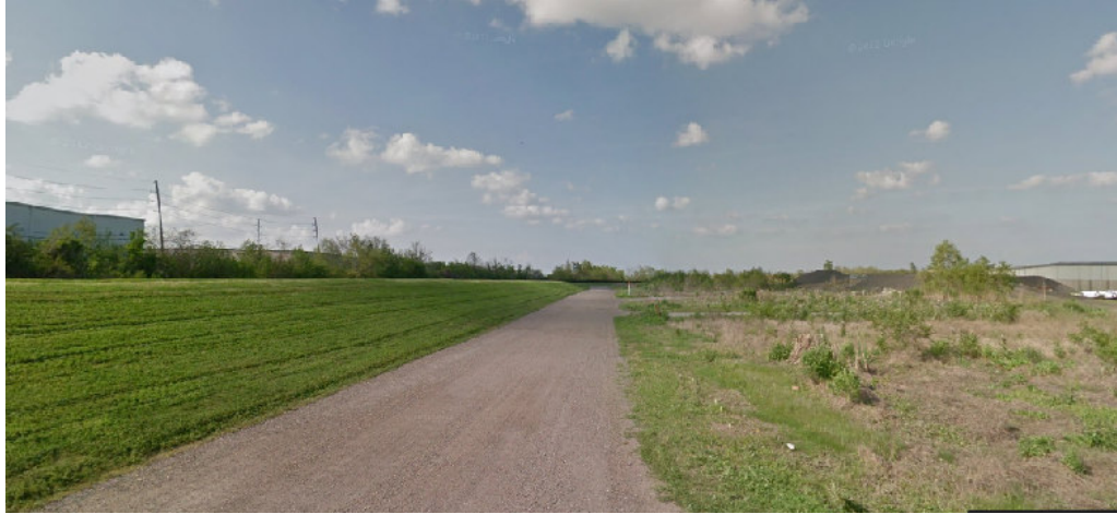
a. Looking North from Near North End of Dixieland Drive, Levee/Sheet Pile
