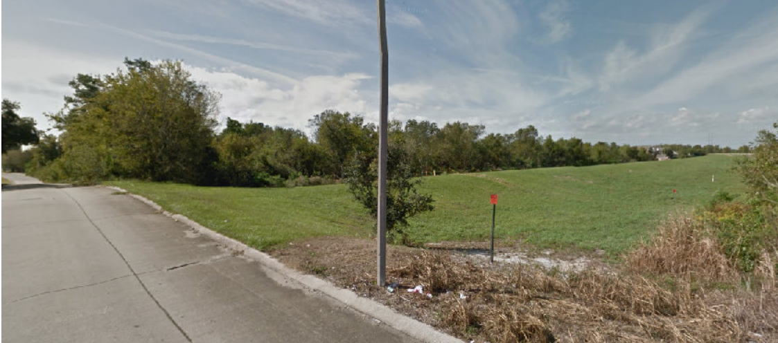
Figure 7.7. Maxent Levee, Looking East at Michoud Blvd Google Earth
