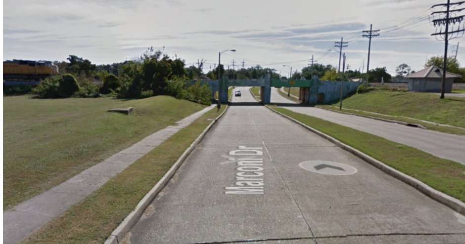
Figure 7.6. Marconi Drive Underpass of NS Railroad Google Earth
