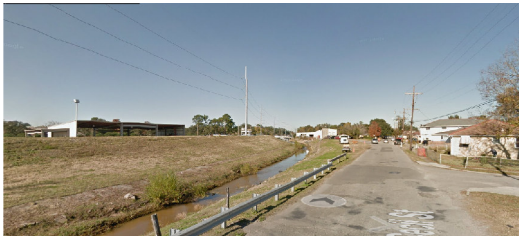
h. Looking North, from Airline Hwy, Levee
