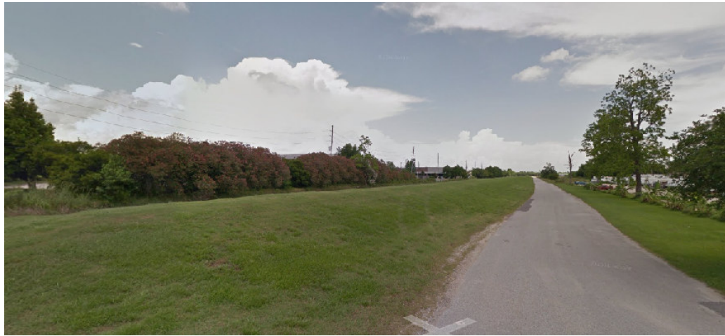
b. Looking North from Airline Hwy, Levee
